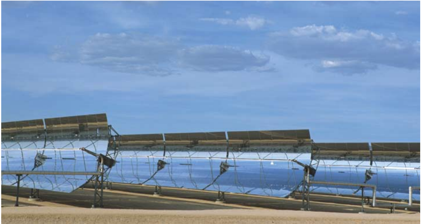
Figure 1 | A parabolic solar collector focuses the sun's energy onto a receiver pipe containing a heat transfer fluid to generate steam used to produce electricity. [Courtesy of Solutia Inc.]
